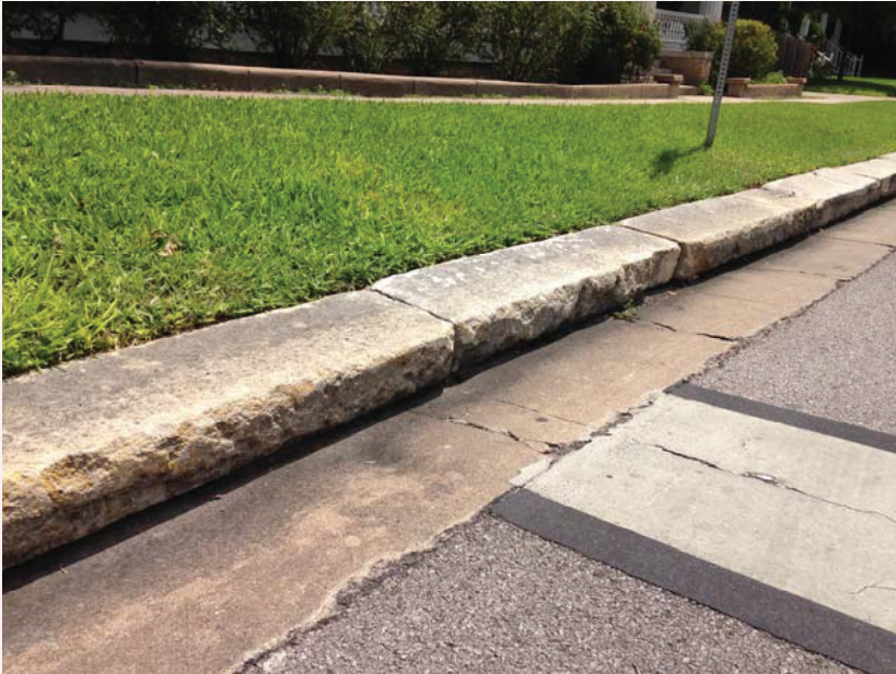
STONE CURB WITH GUTTER
