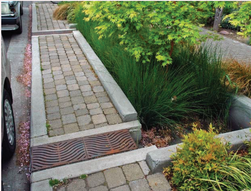
STRUCTURED RAIN GARDEN
