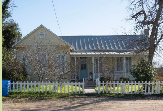
Resource 31A - McClendon House/ Telephone Exchange
