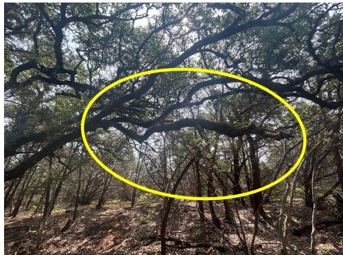
Photo 9. A large live oak was found with tearing cuts on two dead branches. These branches should be cut back to the live stem with a proper pruning cut. The pruning cut should be painted.
