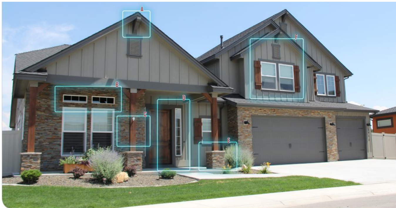
» This single family residential home has a number of added architectural elements including: {A} corbels to emphasize roof gables; {B} transom windows to create more interest; {C} stained wood columns and accents, to frame the entry and front of the house; {D} sidelights to emphasize the entry; {E} stone column bases with caps to anchor the building; and {F} shutters and trim around windows and vents to accent and transition materials.
