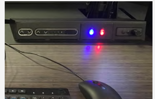
Operators control the PCS with a single-touch switch.
