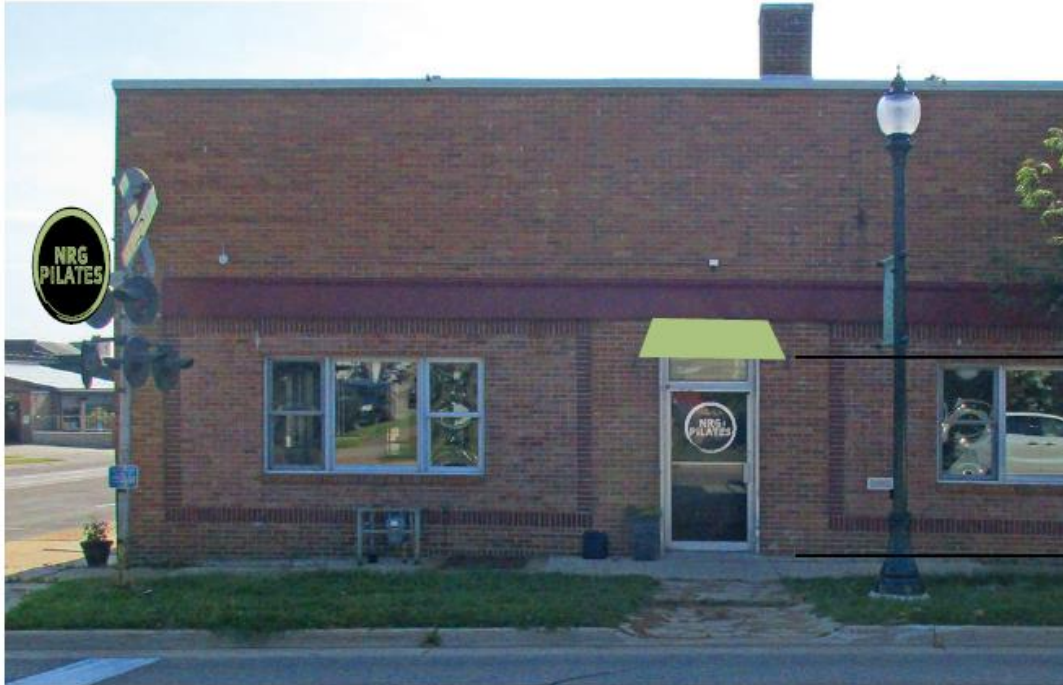
AWNINGS & PROJECTION SIGN TO BE INSTALLED WITH WEJIT ANCHORS AND EPOXY IF NEEDED
