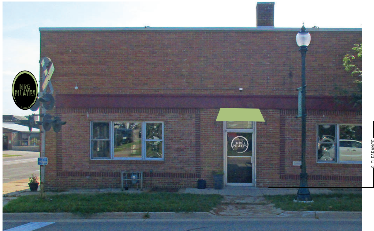
AWNINGS & PROJECTION SIGN TO BE INSTALLED WITH WEJ-IT ANCHORS AND EPOXY IF NEEDED
