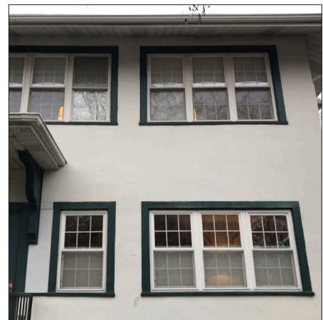
Stucco building FACADE.
