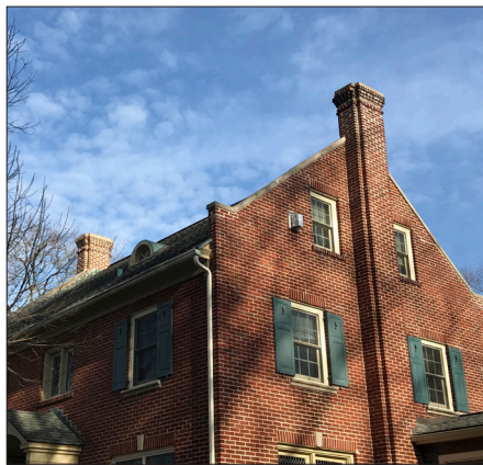
Parapet wall as Dutch Gable
