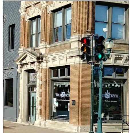
Ground STORY SHOPFRONT and upper story double-hung windows
