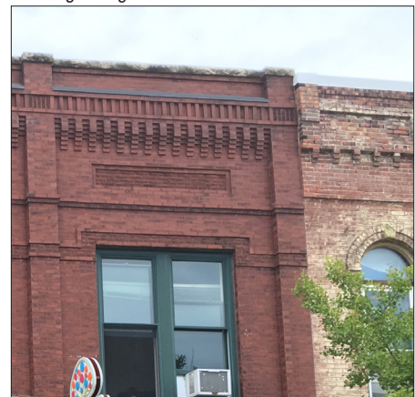
Parapet walls with projecting brick corbels
