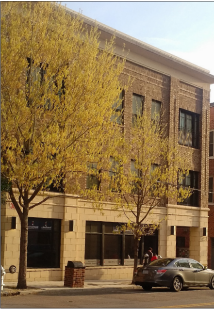
Building with stone and brick FACADE
