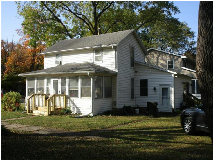
Figure 2 - Existing House On Property
