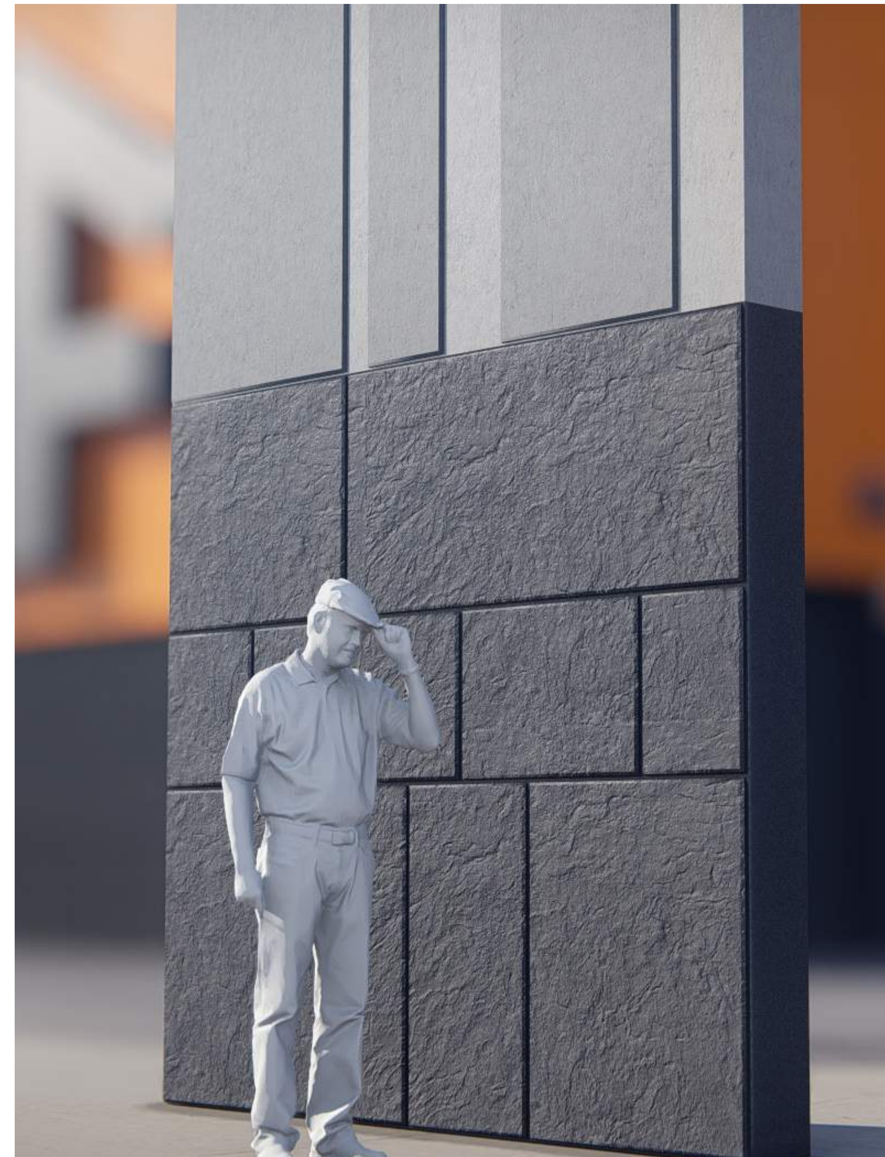
Typical Precast Panel
