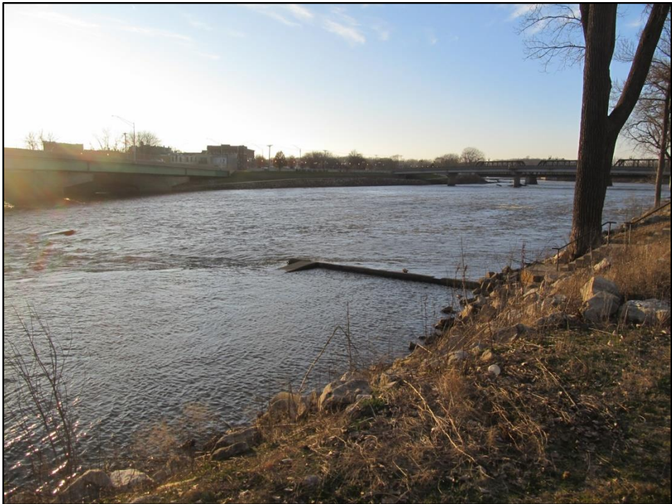
A view of the Clay Hole and remaining portion of the low head dam
