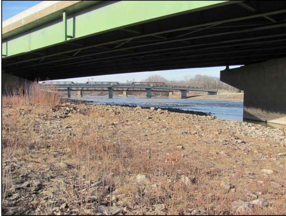
View of the riverbank at the 1 st Street Bridge
