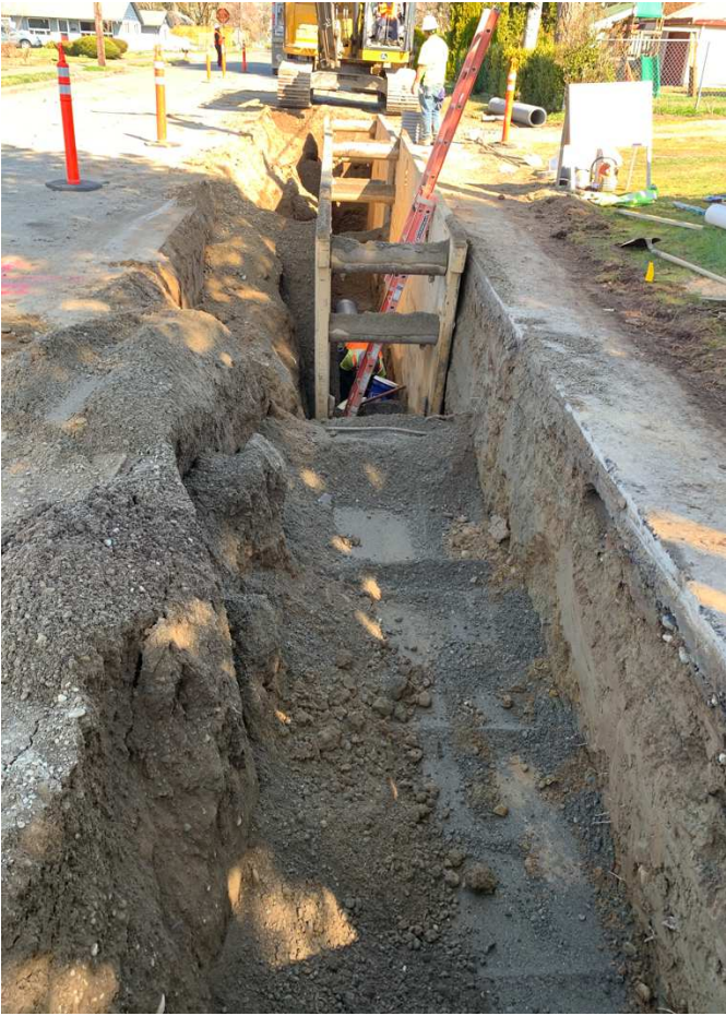
November 14, 2022 – Crossing Sheridan Road with new storm main.
