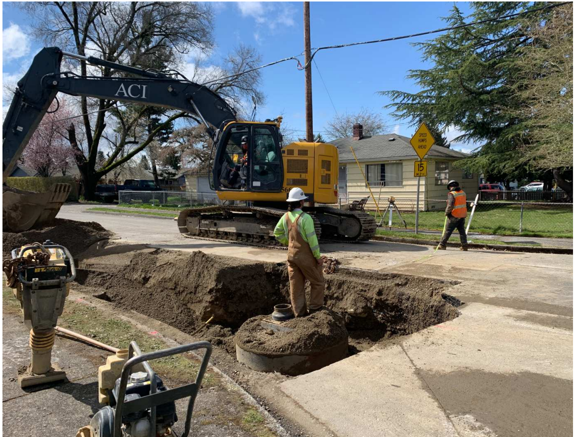
April 7, 2023 – Installation of catch basin on Robin Avenue south of Dibb Street.
