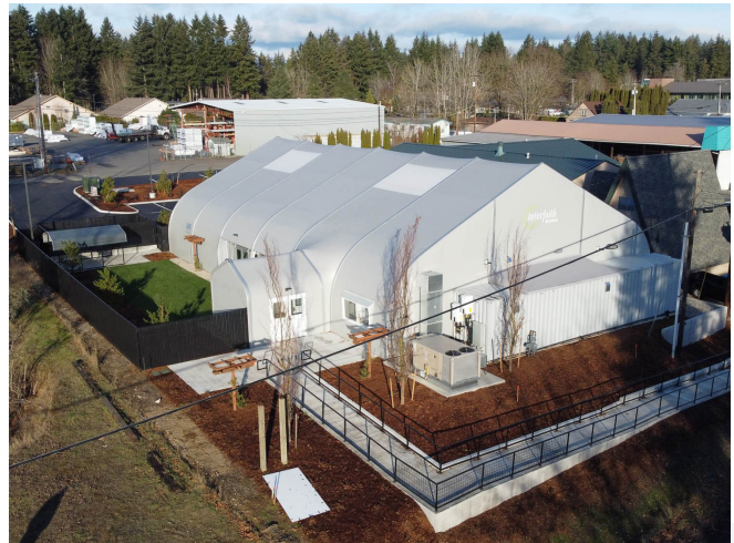
Sprung Shelter, Washington
