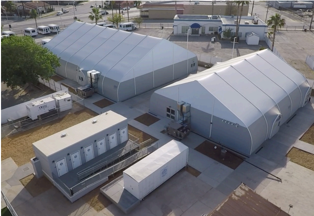
Sprung Shelter, Washington
