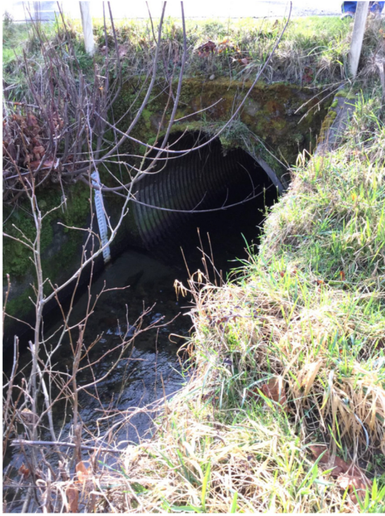
Graphic 2. Existing Culvert Outfall (48" CMP)
