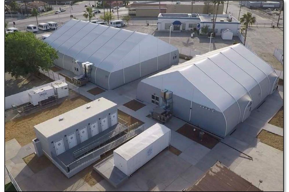
Sprung Shelter, Washington
