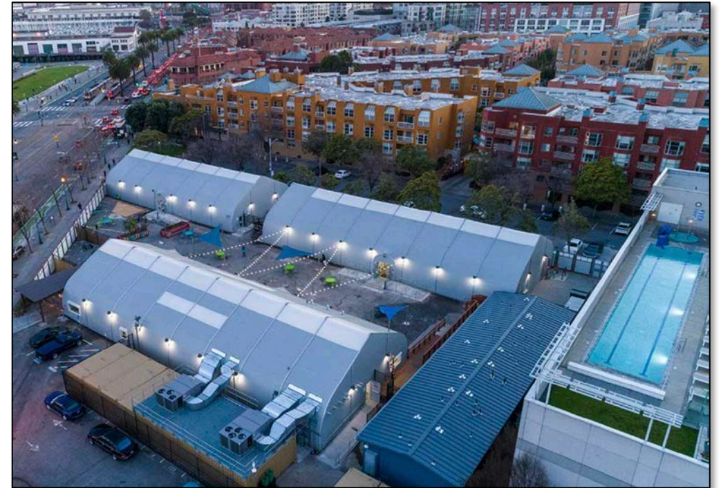
Sprung Shelter, California
