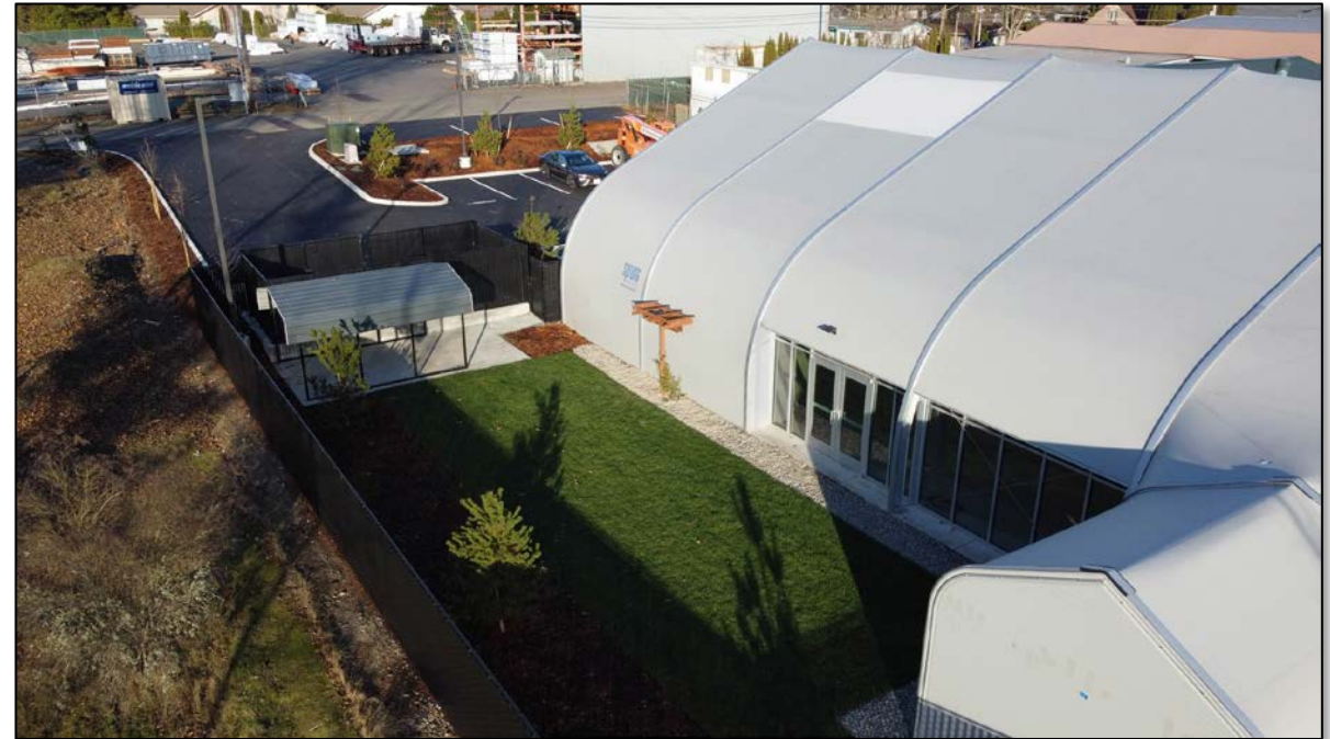
Sprung Shelter, Washington
