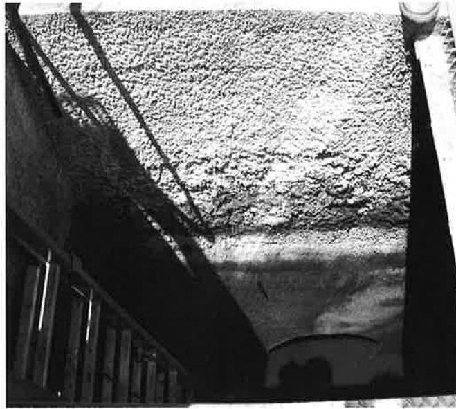
Primary Clarifier 1 Pit
