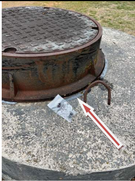
Photograph D-7: Gray/black caulk/sealant (iron to concrete) around top perimeter of manhole riser, west of basin, contains 12% chrysotile ACM, Category I, non-friable in damaged condition. Note that black tar on side of concrete riser and black tar/wrap on nearby pipes do not contain any asbestos.
