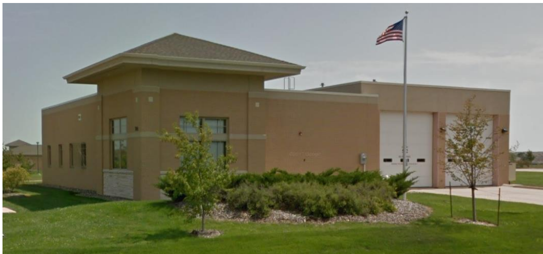
Corner of S. Main Street and Bluebell Road (Cedar Falls Fire and Ambulance Building)
