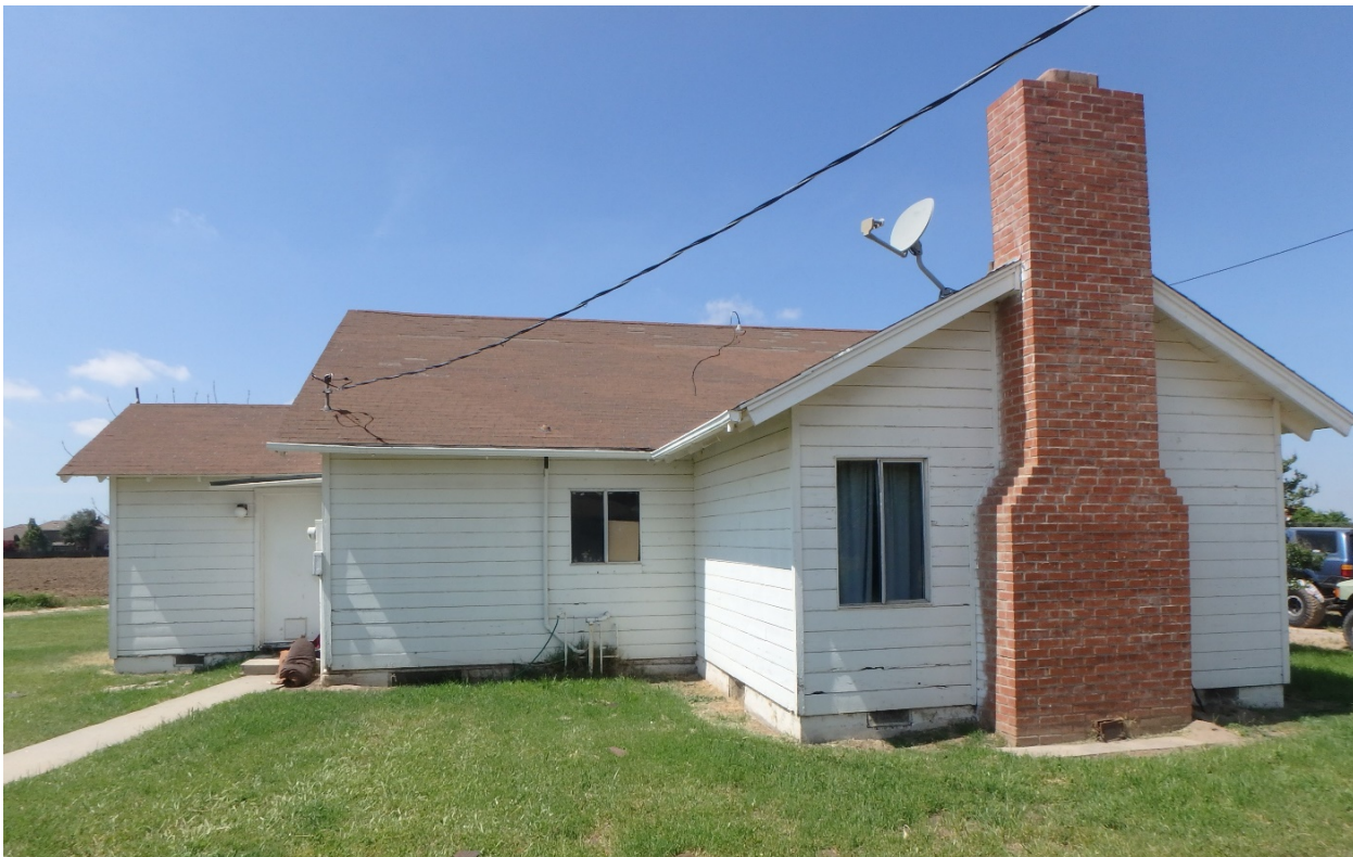
P5b. Description of Photo: East façade with chimney, looking west.
