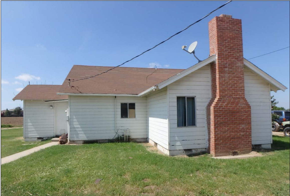
Figure 4-5 East façade of historical dwelling within AE-4027-01, looking west.
