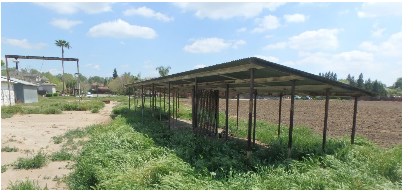
P5b. Description of Photo: Shade structure, looking southeast.
