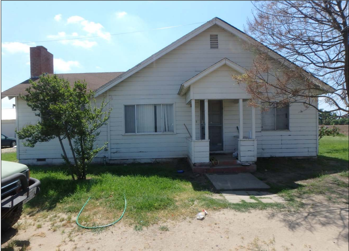
Figure 4-4 North façade (principal face) of historical dwelling within AE-4027-01, looking south.
