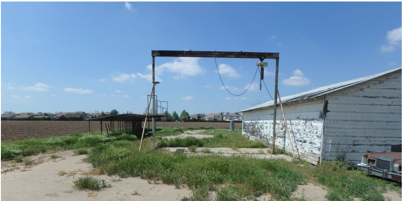
P5b. Description of Photo: Metal hoist and cable winch with concrete pad, looking west.
