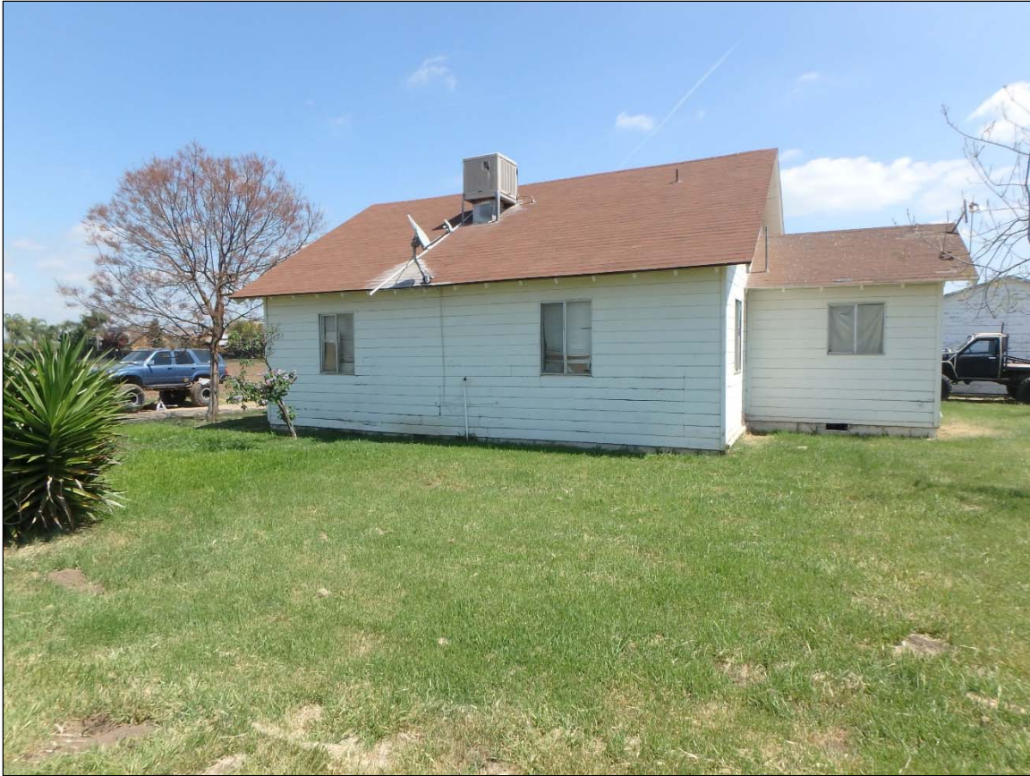
Figure 4-6 West façade of historical dwelling within AE-4027-01, looking northeast.
