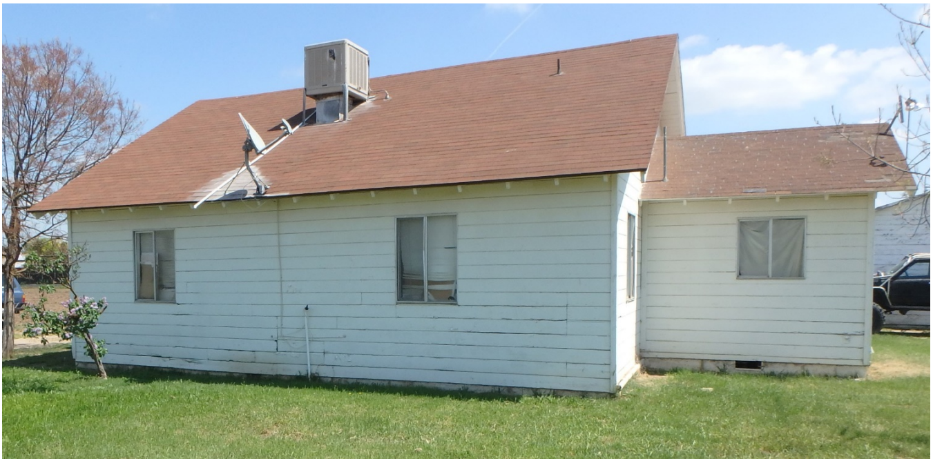
P5b. Description of Photo: West façade, looking east.
