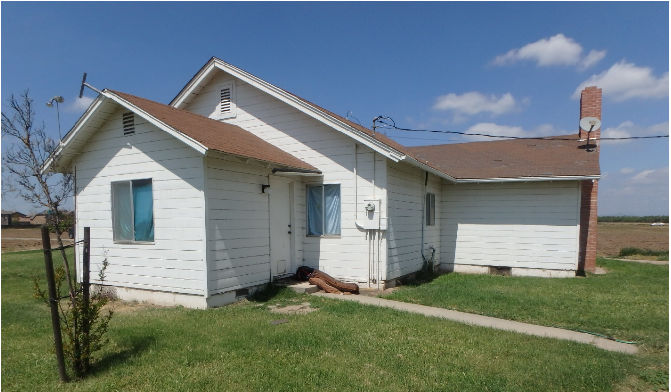
P5b. Description of Photo: South and east facades, looking north.
