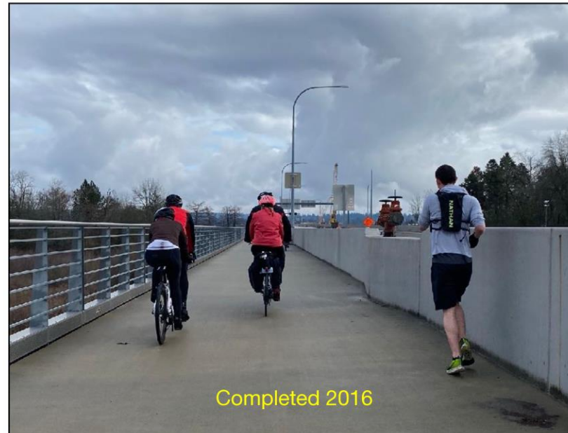
SR-520 Floating Bridge 14-ft shared use path connects Medina to Seattle
