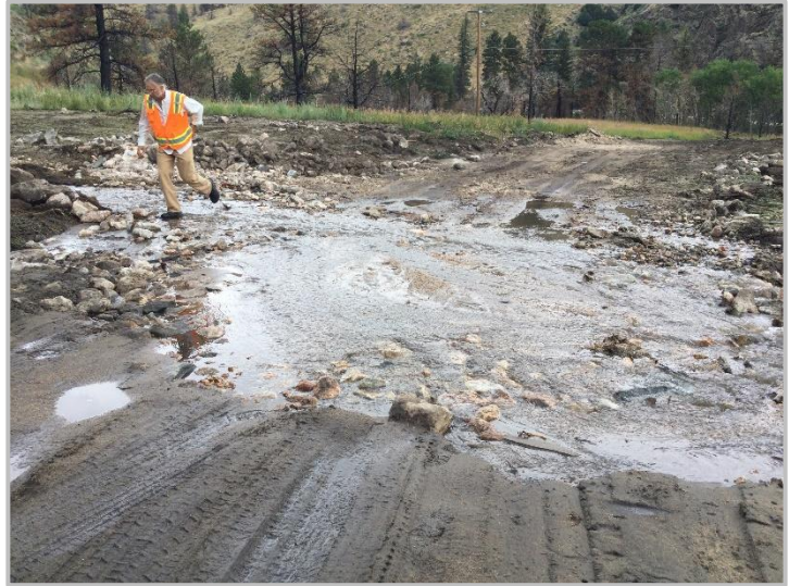
Figure 4: Road damage resulting from increased runoff generate in a post-fire watershed during a 2021 summer storm event.
