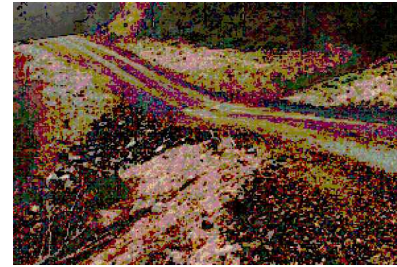
TYPICAL ROLLING DIP ROCK FORD
