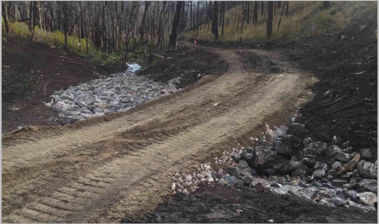
Figure 13: An Armored Drainage Crossing completed at Sheep Creek.
