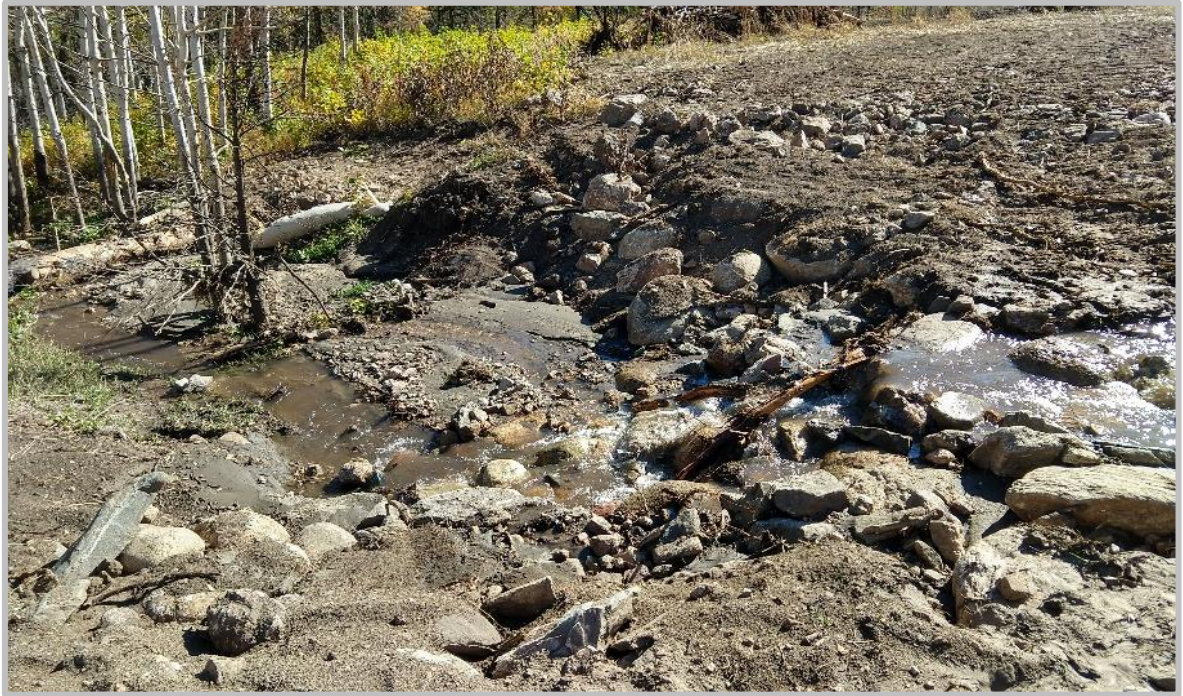
Figure 8: Rock Stabilization downstream of a fire-impact watershed. Installed during 2021 mitigation efforts.
