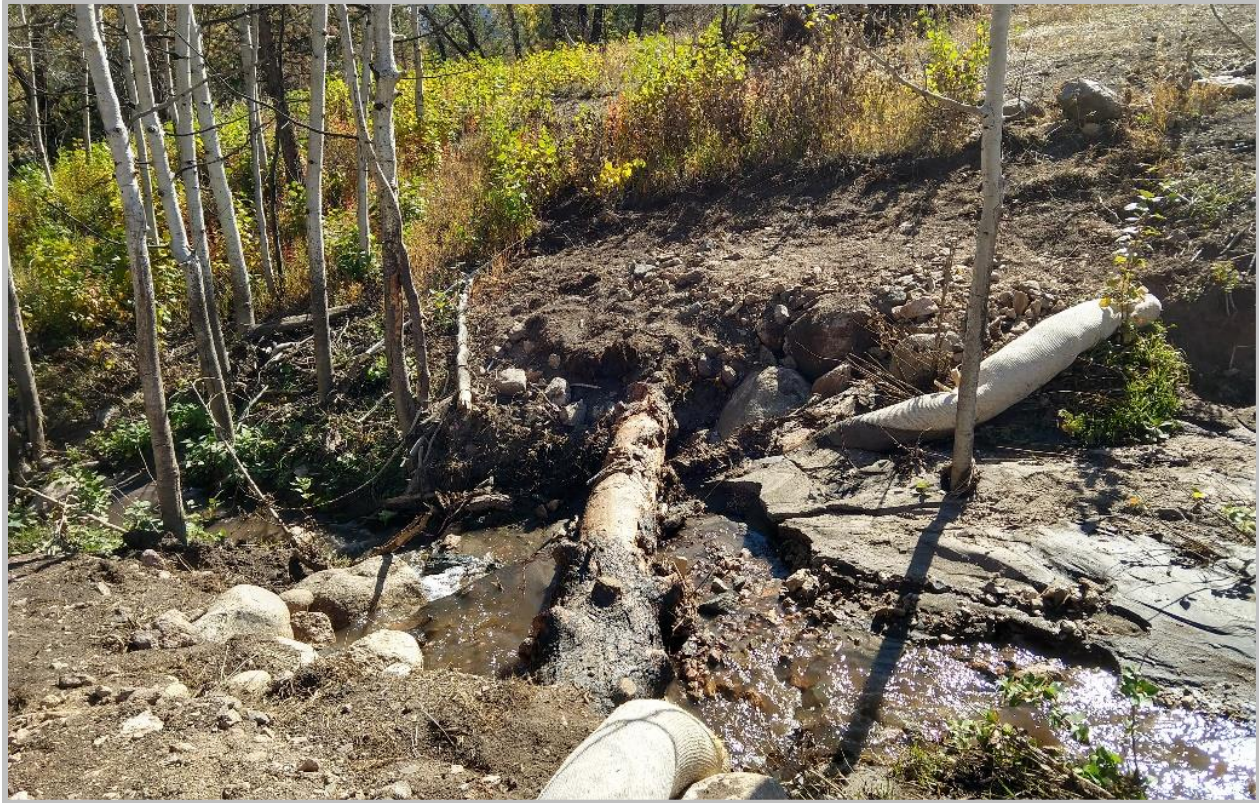
Figure 9: A log jam installed and enhanced with a wattle during Fall 2021 mitigation.
