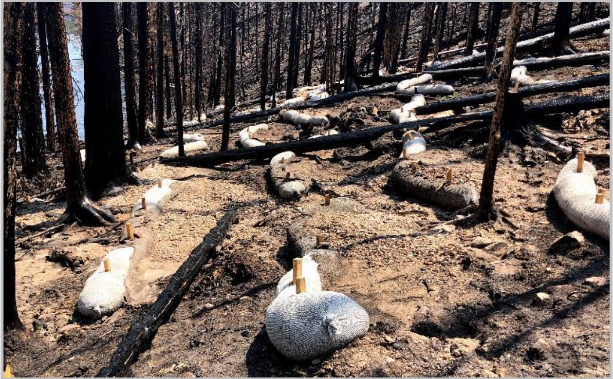
Figure 10: Hillslope wattles creating significant deposition and storage on vulnerable hillslopes just upstream of Chambers Lake.
