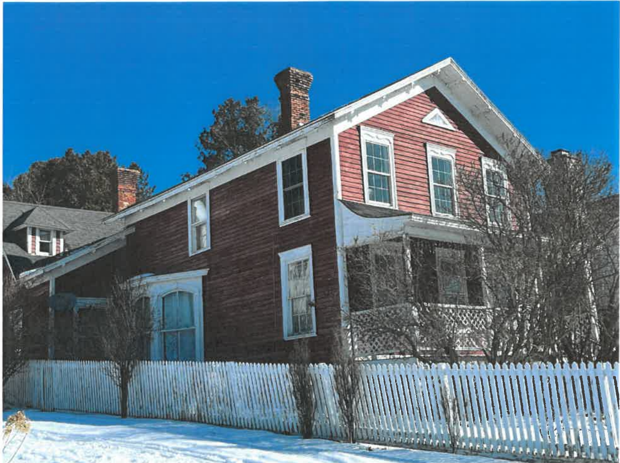
Photo 2. 6948 Main Street, c. 1840.
