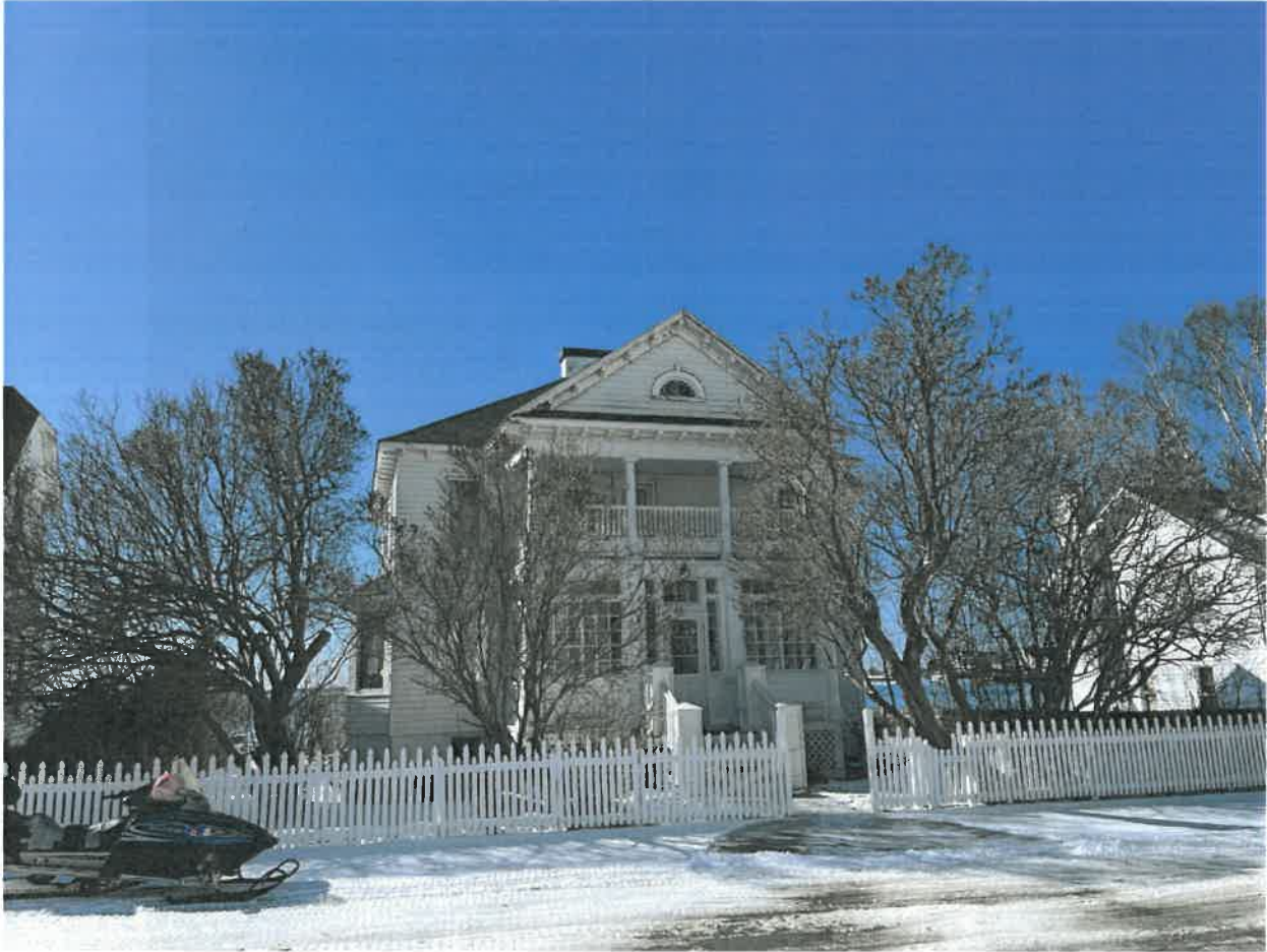
Photo 5. Saint Anne's Rectory, 6837 Main Street
