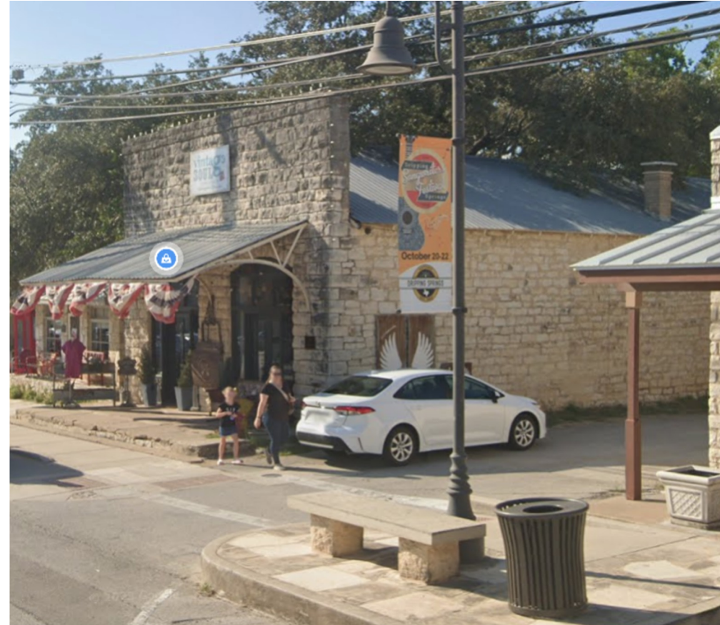
The Mercer Street Historic District uses limestone flagstone paving, limestone benches, specialty pedestrian street-lighting poles and litter bins to enhance the unique identity of this main street.
