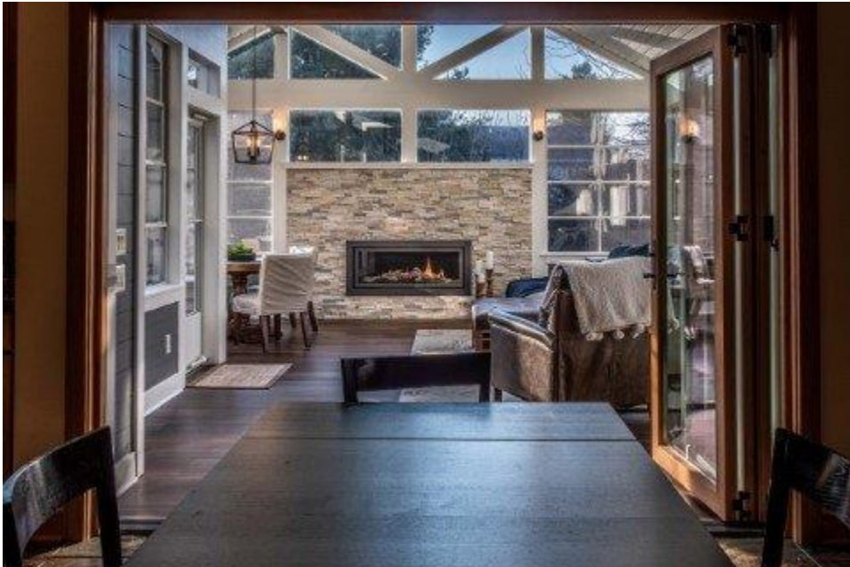
A 3-season room connected to the home with a folding hinged patio door, it uses a gas fireplace for occasional winter heating.
