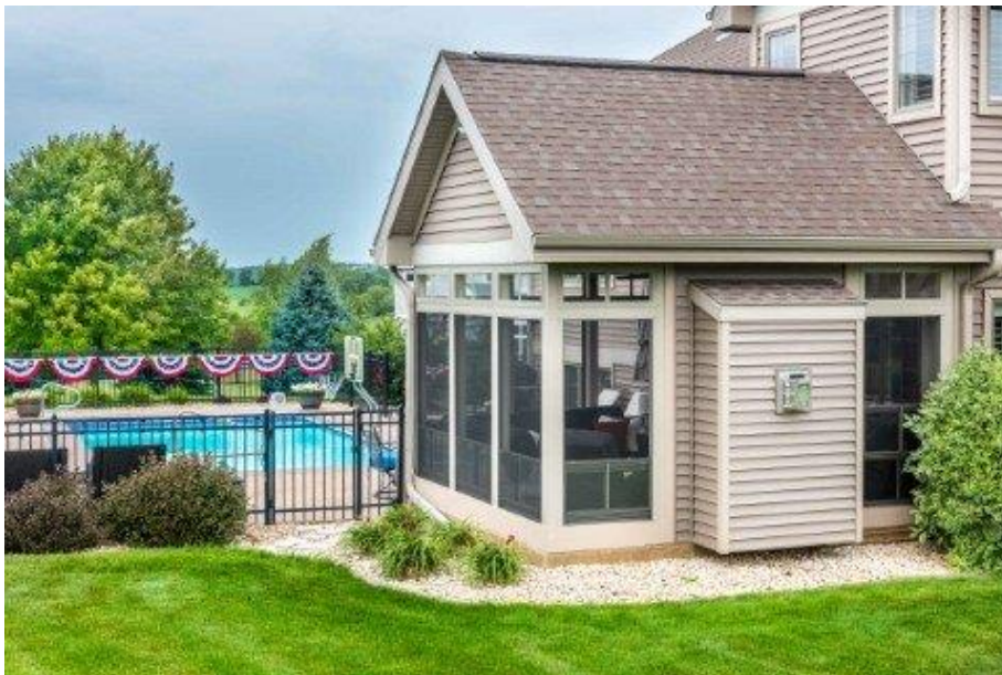
This screened porch was converted to a 3-season room with a fireplace, the perfect way to enjoy the pool and backyard view!
