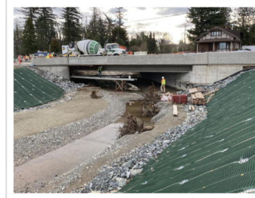
Main Street Bridge
