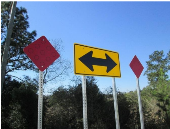
FIGURE 4-23. END OF ROADWAY (TYPE 4 OBJECT MARKER) AND DOUBLE-HEADED ARROW SIGNS TO BE USED IF SANDHILL ROAD APPROACH IS CLOSED OFF
