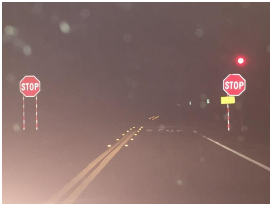
FIGURE 4-5. VIEW OF PAVEMENT MARKINGS, SIGNS AND RPMs ON MARLOW ROAD AT STUDY INTERSECTION DURING NIGHT INSPECTION
