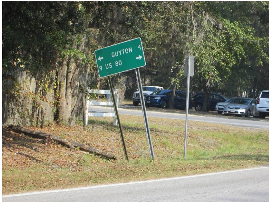
FIGURE 4-8. DAMAGED DIRECTIONAL SIGN ON NORTH SIDE OF SANDHILL ROAD APPROACH (NORTHWEST QUADRANT OF STUDY INTERSECTION)
