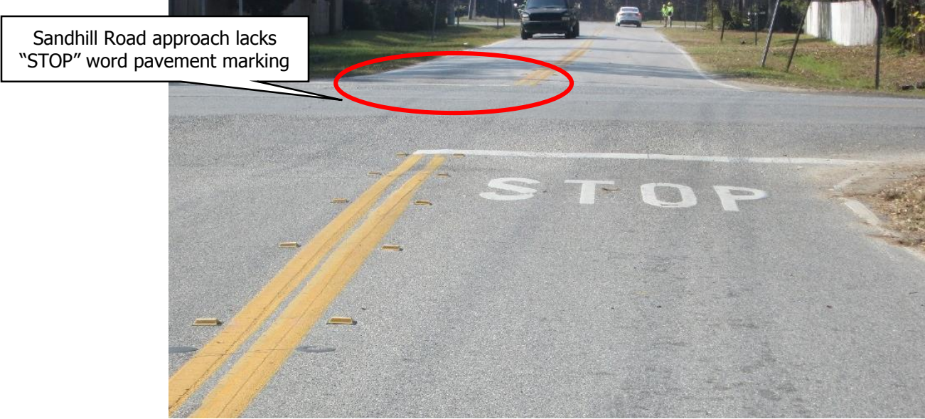
FIGURE 4-3. VIEW OF PAVEMENT MARKINGS AND RPMs ON MARLOW ROAD AT STUDY INTERSECTION
