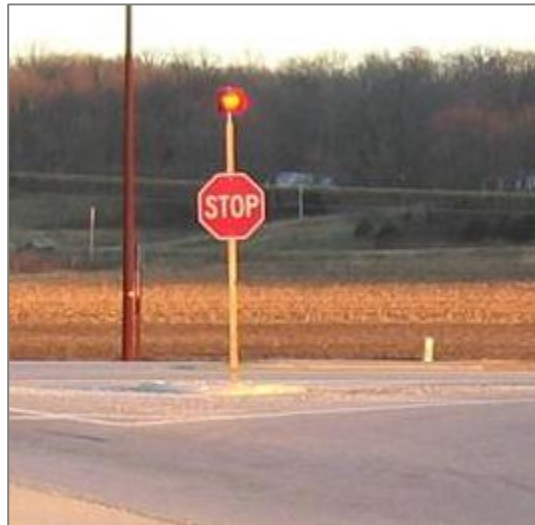
FIGURE 4-15. EXAMPLE OF A FLASHING BEACON MOUNTED ON A "STOP" SIGN. SOURCE: FHWA PUBLICATION HRT-08-044 3
