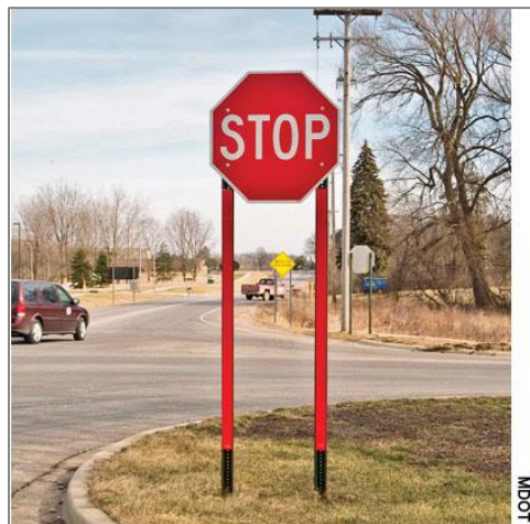
FIGURE 4-13. DOUBLE-POSTED STOP SIGN WITH REFLECTIVE STRIPS ON THE POSTS. SOURCE: MICHIGAN DOT VIA FHWA 2
