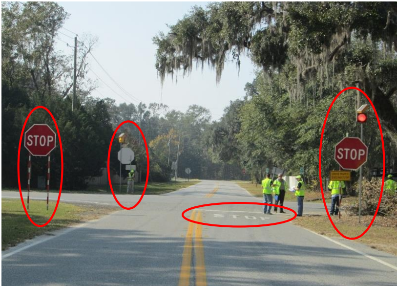
FIGURE 4-1. VIEW LOOKING ALONG WESTBOUND MARLOW RD TOWARD INTERSECTION WITH SR 17. NOTE THE RECENTLY INSTALLED OVERSIZED STOP SIGNS, SUPPLEMENTAL FLASHING BEACONS, AND PAVEMENT MARKINGS
