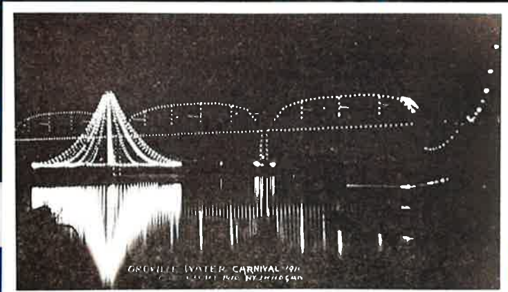
Celebrating completion of the new bridge, Oroville sponsored the first of three water carnivals starting on July 4, 1909. Shown here is a photo taken of the bridge and floats outlined by electrical bulbs at night. (Courtesy, James Lenhoff.)
