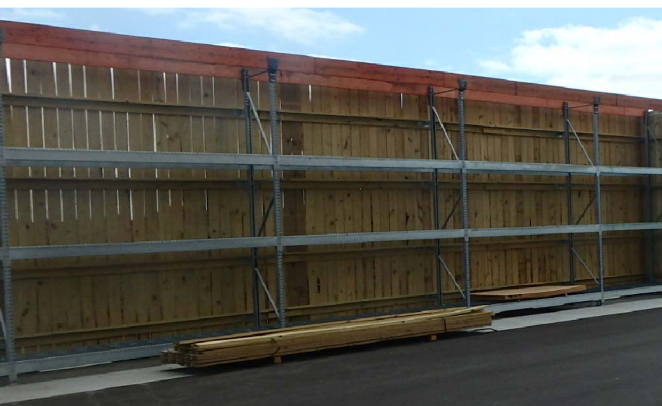
PHOTO OF PERIMETER RACKING/FENCING TAKEN FROM INSIDE YARD
