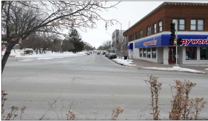
Intersection at 23rd and College Streets: existing pedestrian crossing distance
